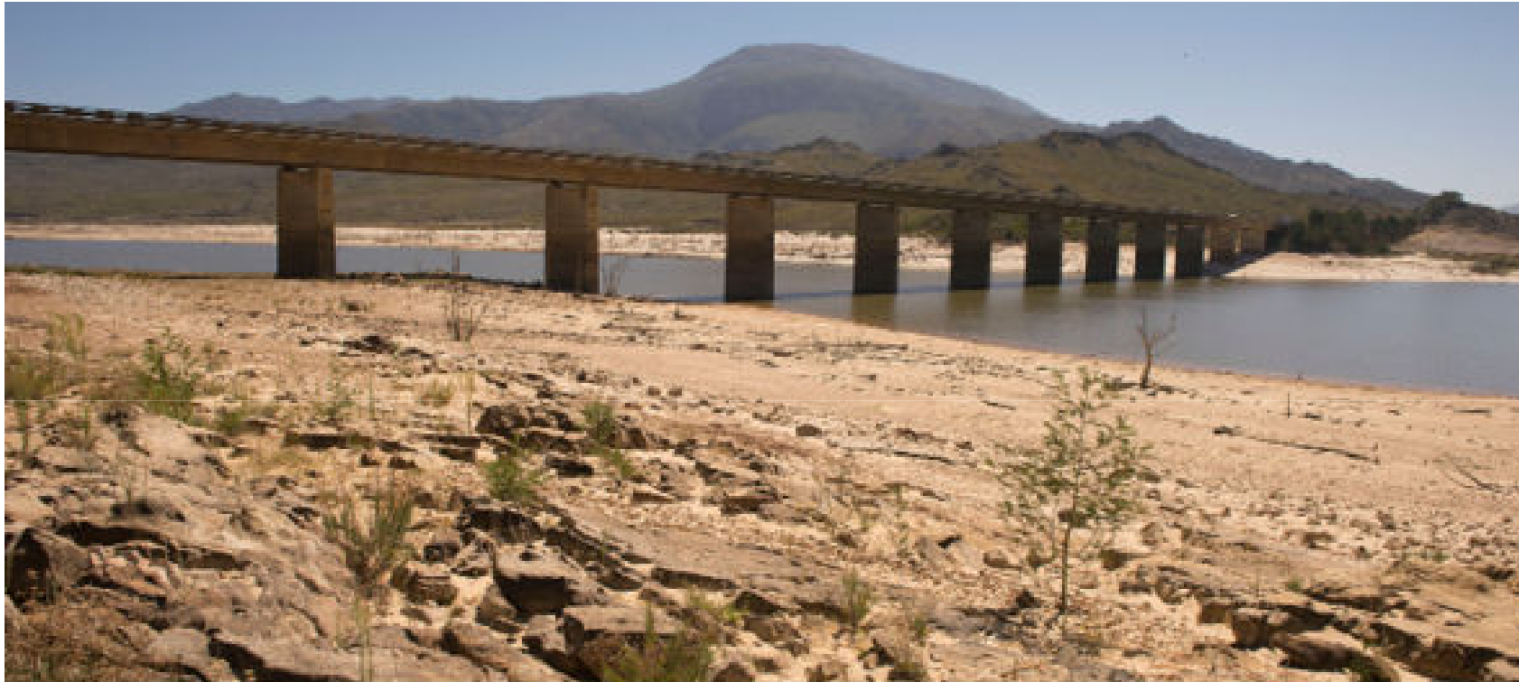
THEEWATERSKLOOF DAM - 20 JAN 2017
