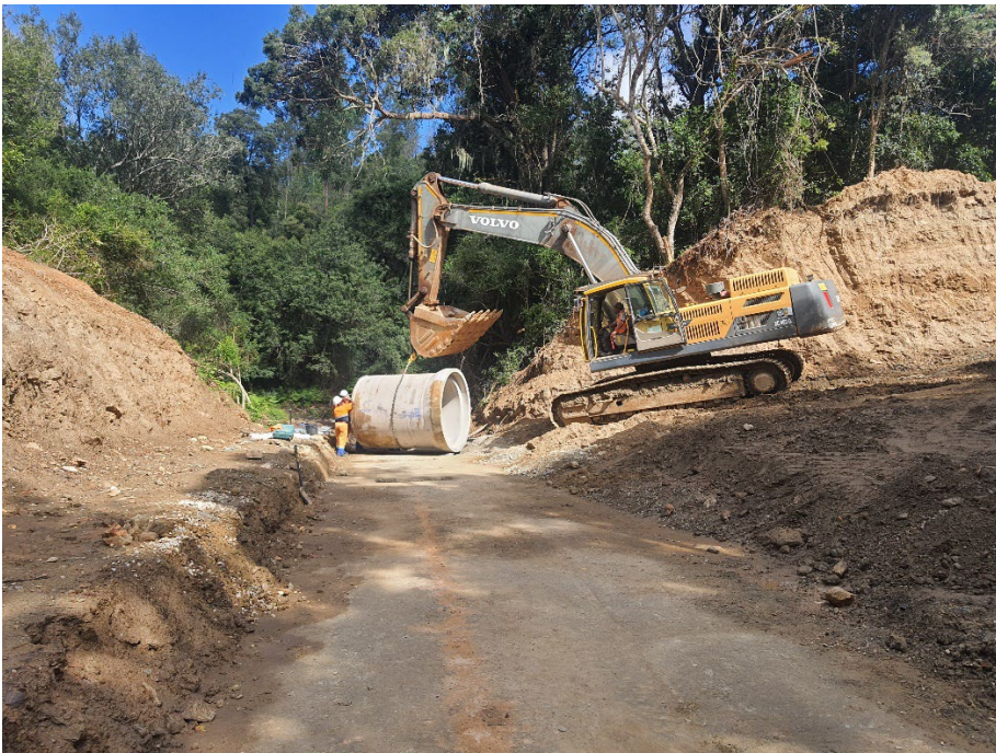
Figure 6: Installation of the 1st pipe
