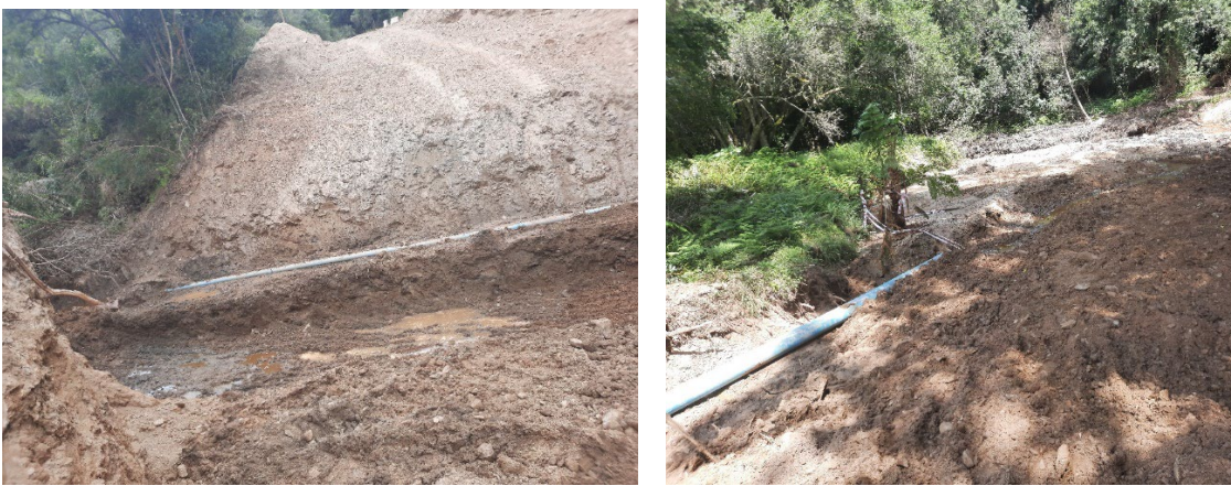
Figure 5: showing excavation and laid PVC pipes
