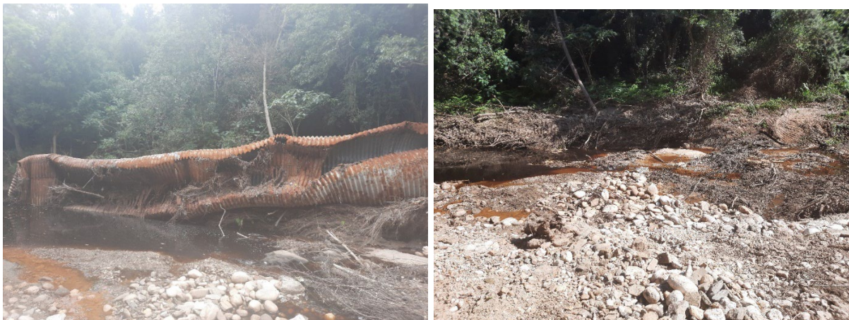
Figure 4: showing the armco and after it was removed
