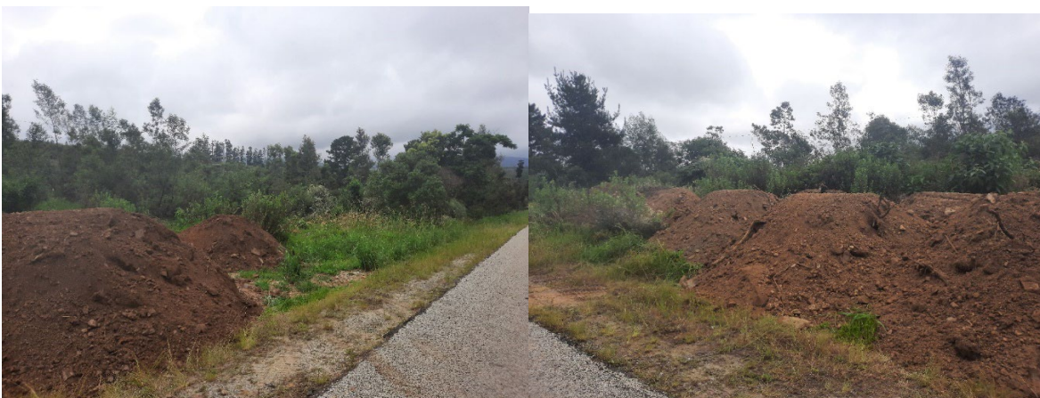
Figure 6: showing stockpiling along the road reserve
