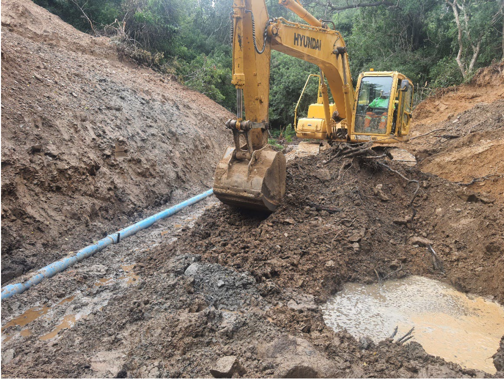
Figure 3: 200mm By-pass pass
