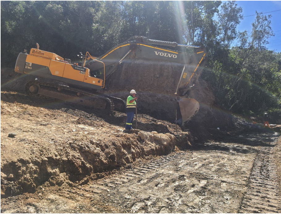
Figure 5: Gravel material with cement
