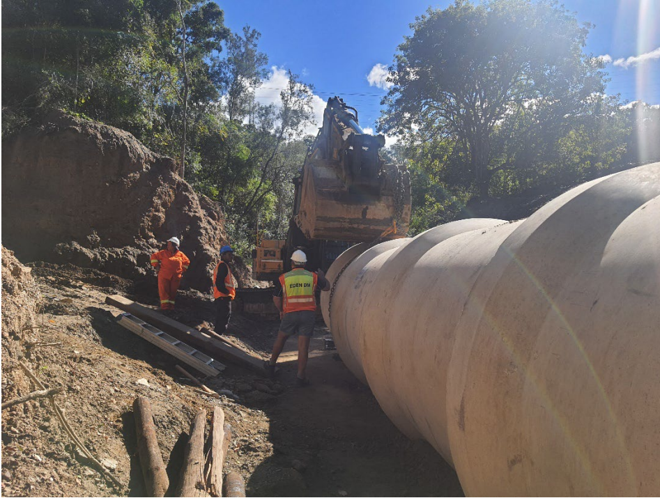
Figure 7: 4th Pipe Installation
